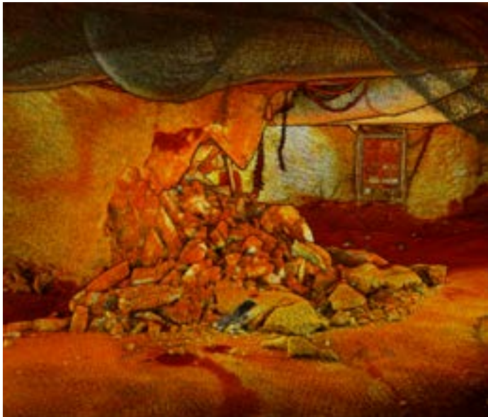
The seismic event triggered rock bursts across kilometers of drifts. Armed with accurate 3D datasets, LKAB engineers were able to start planning remediation work within weeks of the event.
